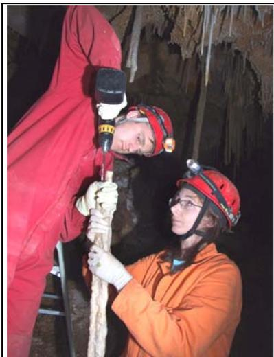
**Enlarging the support pin hole before the final connecting to the roof. Photo by Garry K. Smith**
