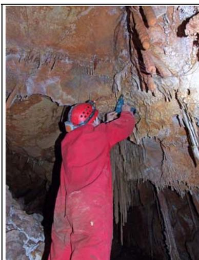
Drilling the attachment point in the ceiling to accommodate the support pin. Photo by GKS.
